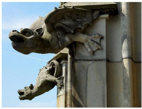
roof. You may have noticed the gargoyles at the four corners of the top of the tower. Through their mouths, rainwater is taken from the tower roof, keeping the roof dry throughout the year. Moss, leaves, etc get washed into the pipes which go through the gargoyles and block them so they have to be cleared from time to time.
